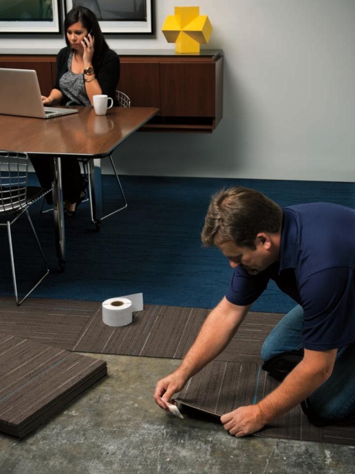
The TacTiles system eliminates the mess, odor and drying time of spread adhesives. With these small, glue-free squares you can install Interface carpet tile with little disruption to normal routines.
