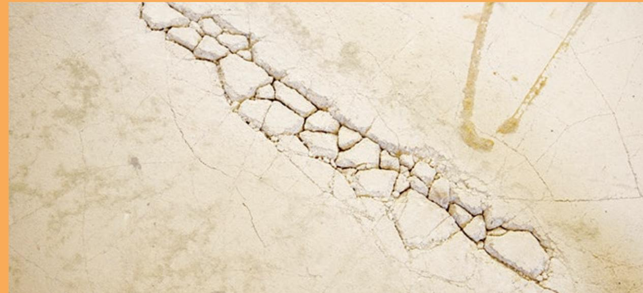
*When you tear out stubborn, glue down broadloom carpet, sections of the subfloor, such as gypsum concrete, can adhere to the back of the flooring and cause much-needed repair before the next flooring installation. Upon repair, switching to a glue-free installation system eliminates this from future floor prep.*
